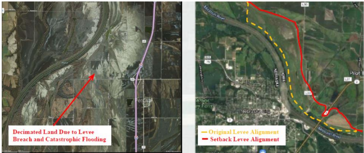
Figure B1; Missouri River Levee L-575 Breach Area and Setback Location
